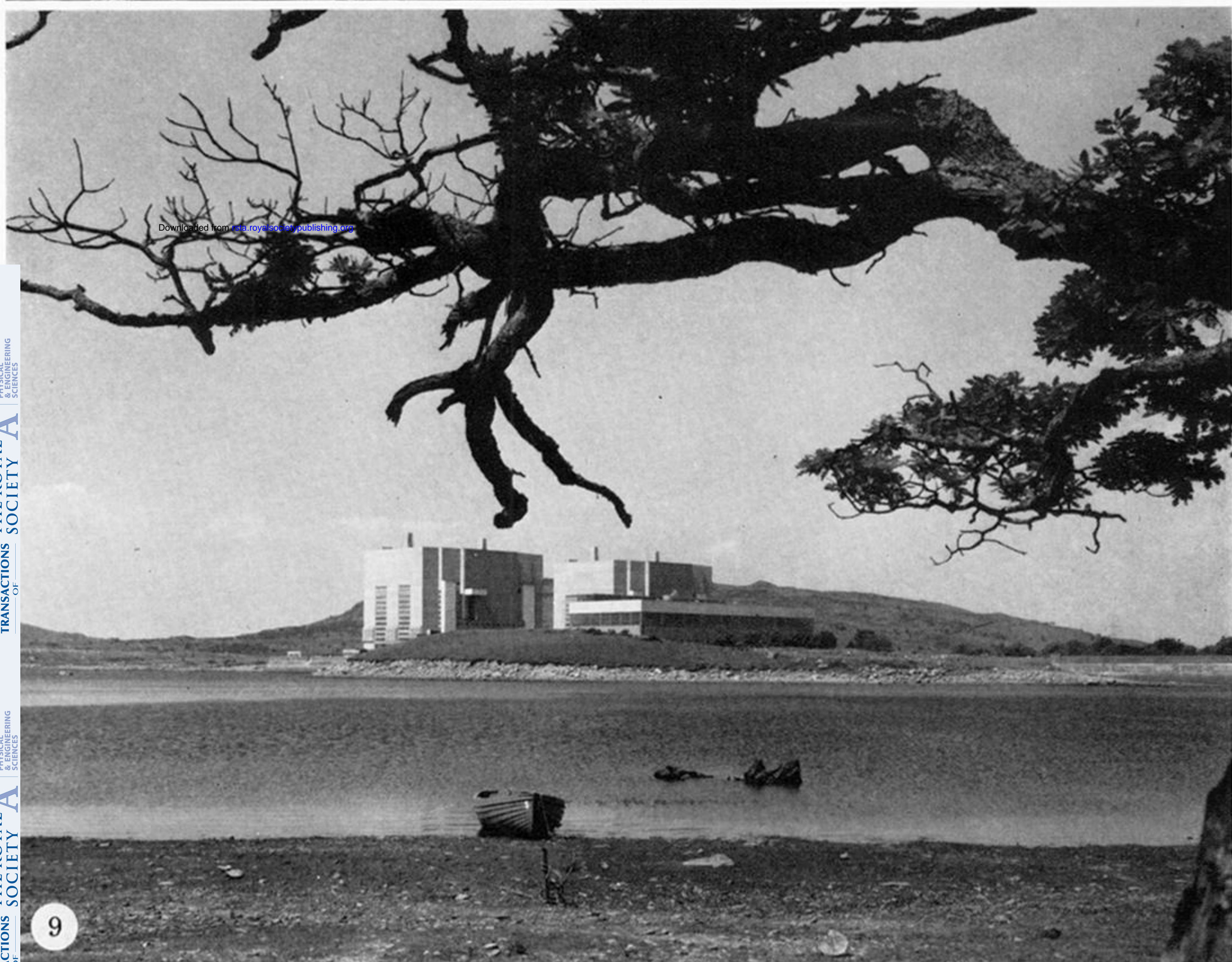
FIGURE 8. Ffestiniog pumped storage station. FIGURE 9. Trawsfynydd nuclear power station.
